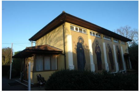
St. Silouan's church
