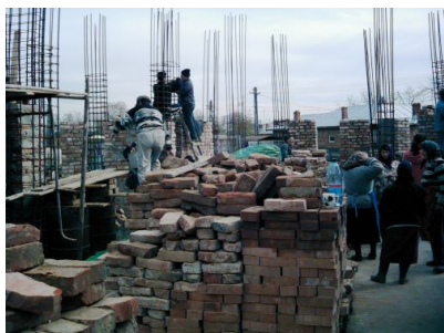
Parishioners working on the site
