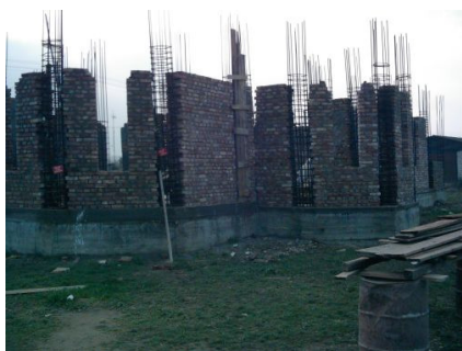
The building site
