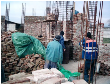
Parishioners working on the site
