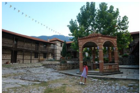
The central courtyard
