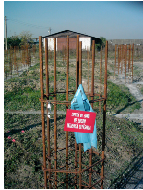
The foundations of the Church have been laid.
