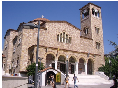
The exterior of the church of St. John
